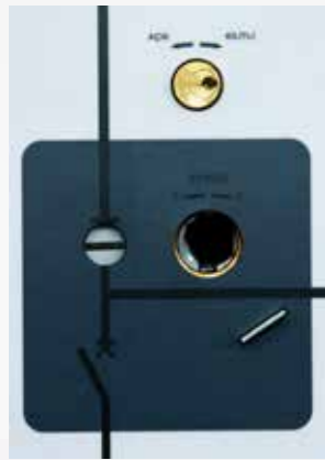
Mechanical interlocking system between disconnect and the circuit breaker to ensure safe maneuvering and to prevent incorrect maneuvering during the work on the line.
