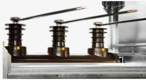
30x10mm dust-resistant main busbar set and field regulators.
