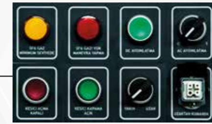
Operator friendly remote control sockets, buttons and signal lamps.
